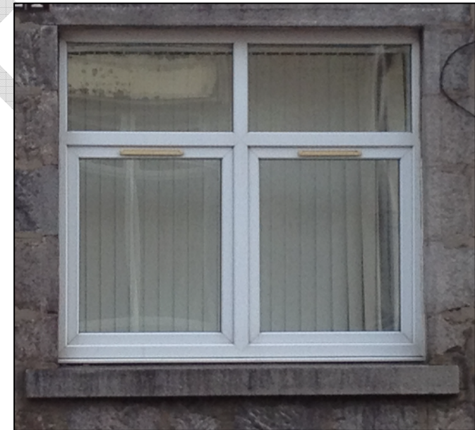
Discreet means of achieving ventilation will be required for Listed Buildings and on public elevations in Conservation Areas
