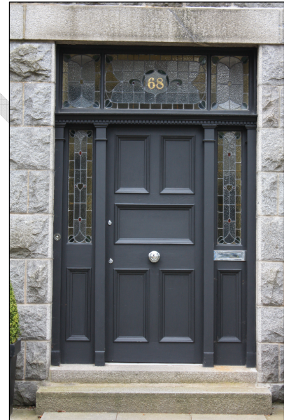
Historic glass should be reused where this contributes to the character of a building
